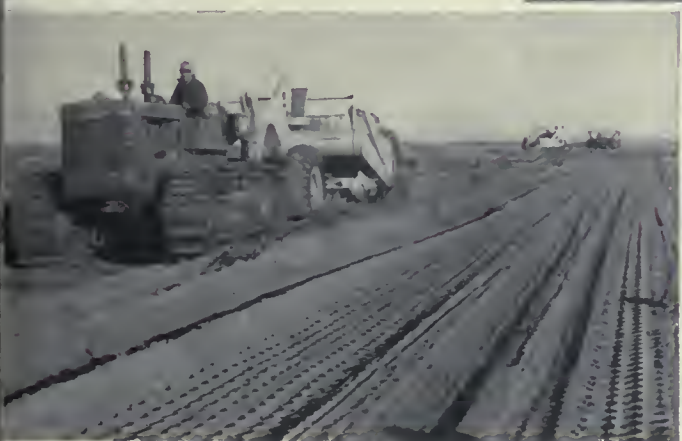
HOW MUCH WILL IT COST TO DEVELOP? —The amount of investment for such items as leveling and with carryalls on the Columbio Bosin project (below) has to be figured in selecting land to be irrigated. Irrigable lands of the Posco Unit, of Mt. Photo below by F. B. Pomeroy, Region 1 photographer, at right by H. C. Robinson, former Region 1 photographer.
